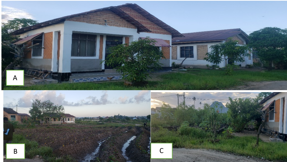
Plate 2: A) Finished and arranged houses for resettlers at Chamazi; B) Vacant land for the affected people who managed to get plots waiting for the NGOs and CBO to have their homes; C) Building foundations of the affected people who are in the process of building their homes, Source: Survey data from Chamazi, 2024
