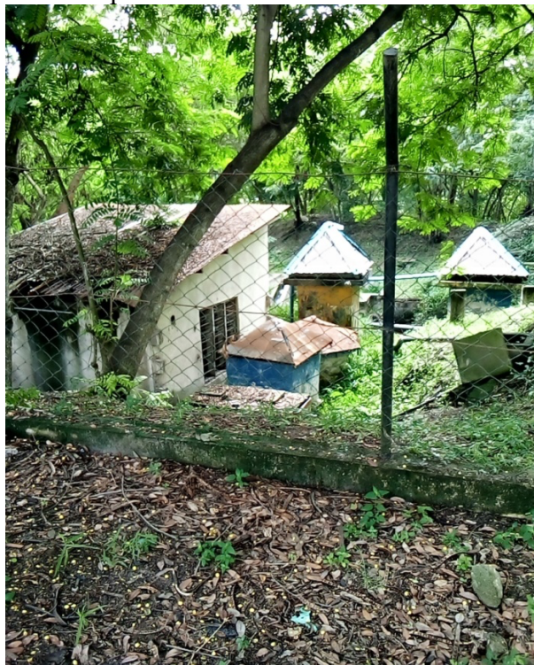
Plate 1: Wastewater Treatment Plant at ARU, Dar es Salaam, Tanzania
