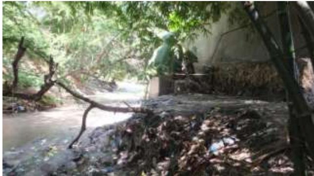
**Plate 7: Blockage of a natural drainage channel as a result of a fence wall that was built on the channel**
